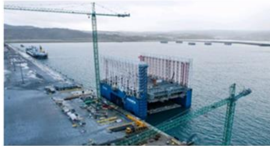
Floating Dock (Reference: Antbuildz | The Construction of Mega Tuas Port)
