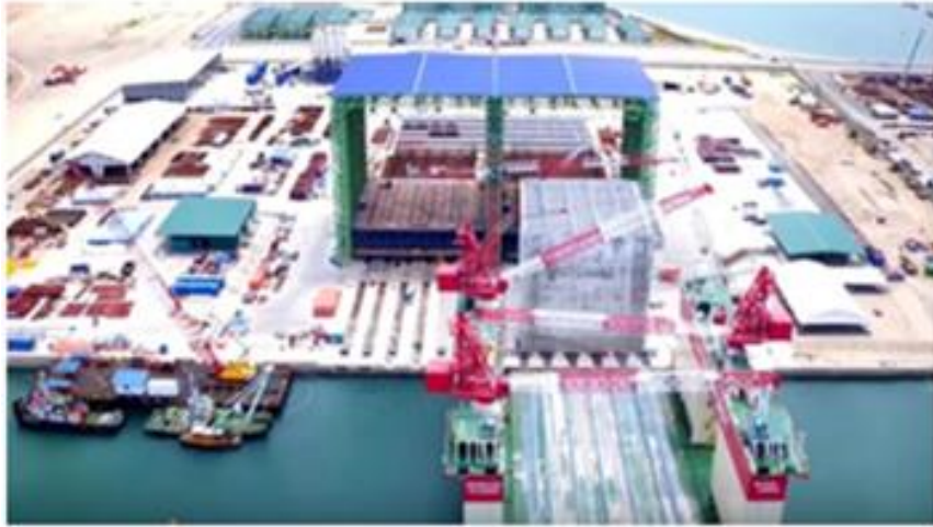
Giant Gantry and moving pre-fabricated caisson to the floating dock (Reference: Antbuildz | The Construction of Mega Tuas Port)
