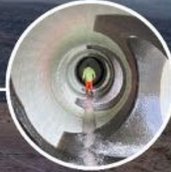
Buried Upper Reservoir
