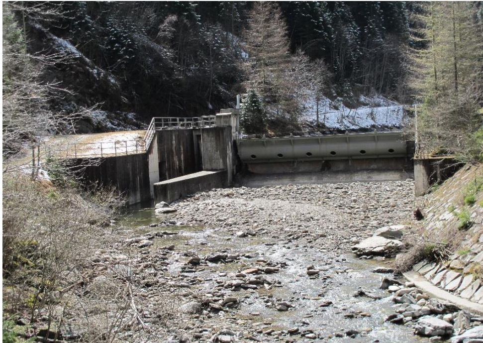
Figure 1. A river is diverted at the weir into a pipeline running under the riverbank on the left side of the picture. The dewatered river reach downstream of the dam is very dry because of low E-flow releases. Such a situation can be avoided by a state-of-the-art E-flow management. Photo: K. Jorde
