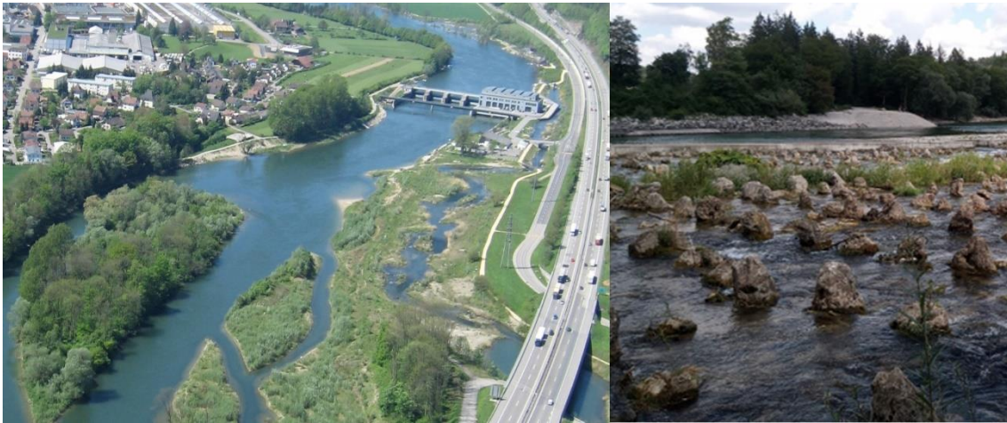
Figure 1. Left: A large-scale nature-like fishway constructed at the Ruppoldingen run-of-river powerplant in Switzerland. On the right side of the powerhouse, a diversion river was implemented for ensuring fish migration (Source: ATEL). Right: The nature-like fishway at Baierbrunn in southern Germany illustrates how a well-designed structure can be integrated into the cultural landscape, providing native fish of different species and life stages an adequate variety of flow conditions for migration, resting, and shelter. (Source: C. Jähnel / University of Innsbruck)
