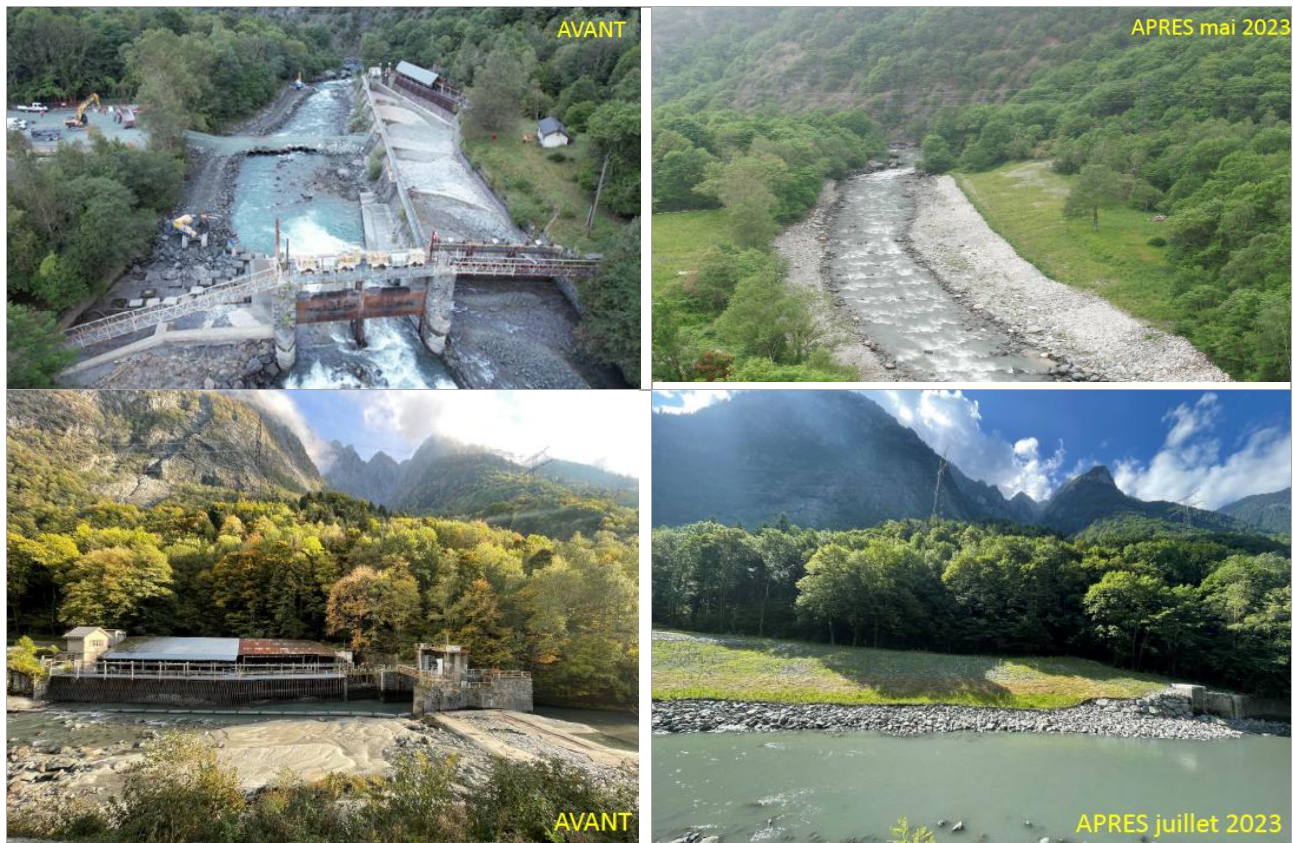
Figure 7.28 Decommissioning of 5 old hydropower plants and renaturation of their sites (©EDF)
