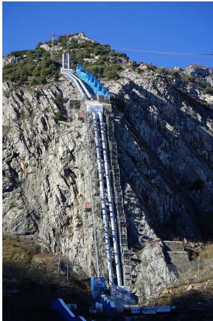
Figure 7.19 Renovation work on the Sabart HPP penstocks (© EDF)
