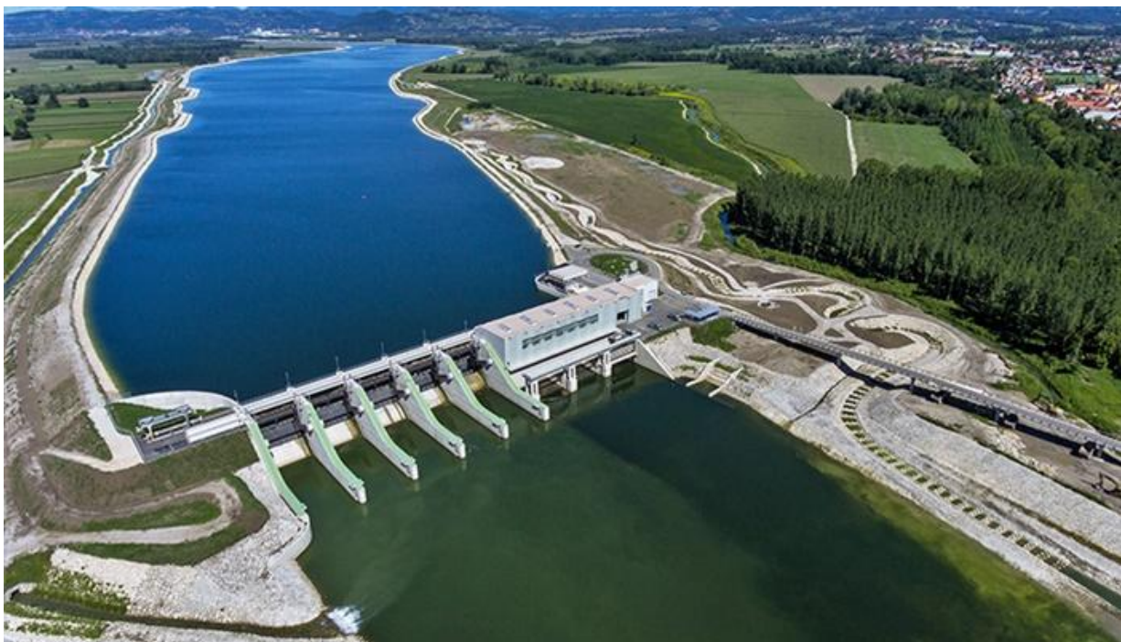
Figure 7.5 Hydropower plant and its fish pass on the Sava River (Energetika.ba)
