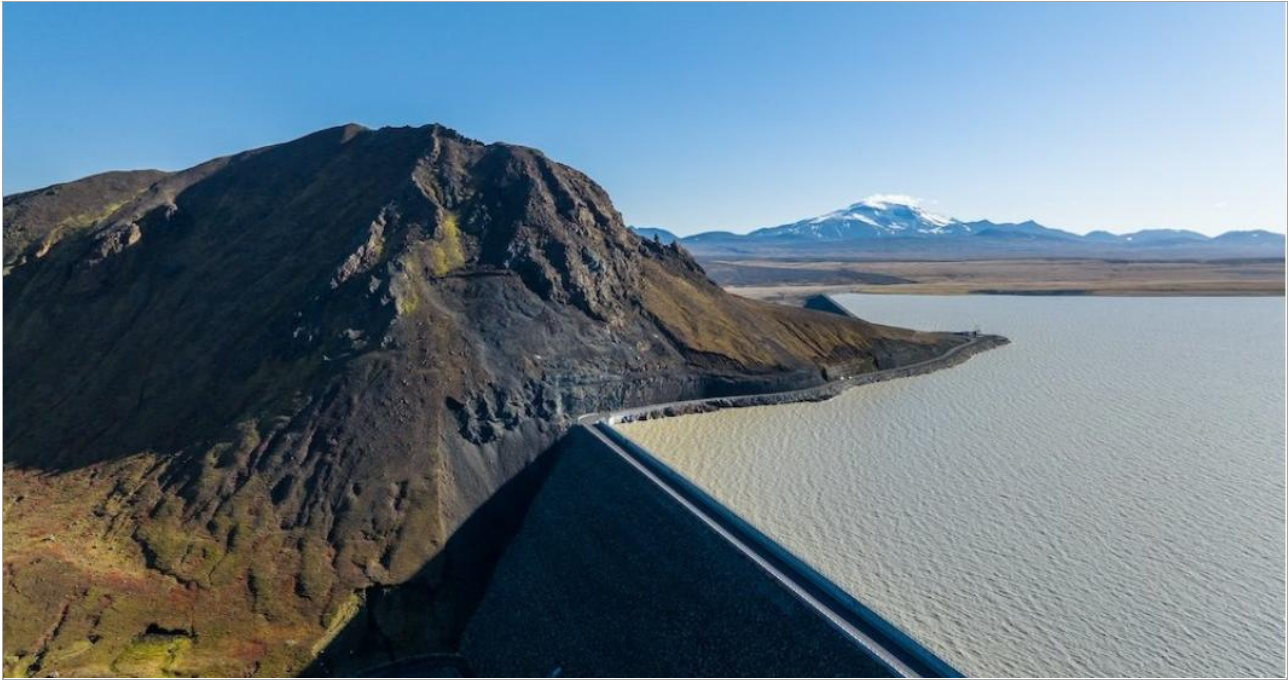
Figure 7.16 Kárahnjúkar Dam (HSA)
