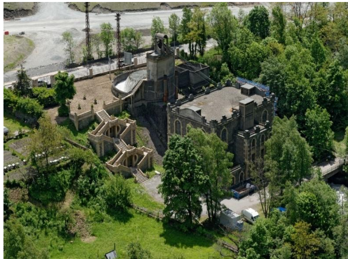
Figure 7.30 The restoration of Les Vernes hydro plant
