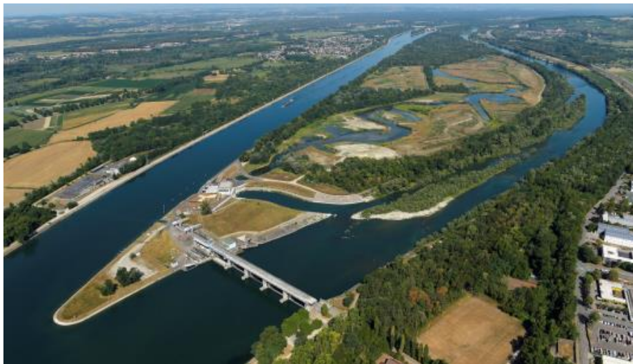
Figure 7.10 The Rhine River, the Kembs dam, Kembs island with the new HPP and river (©EDF)
