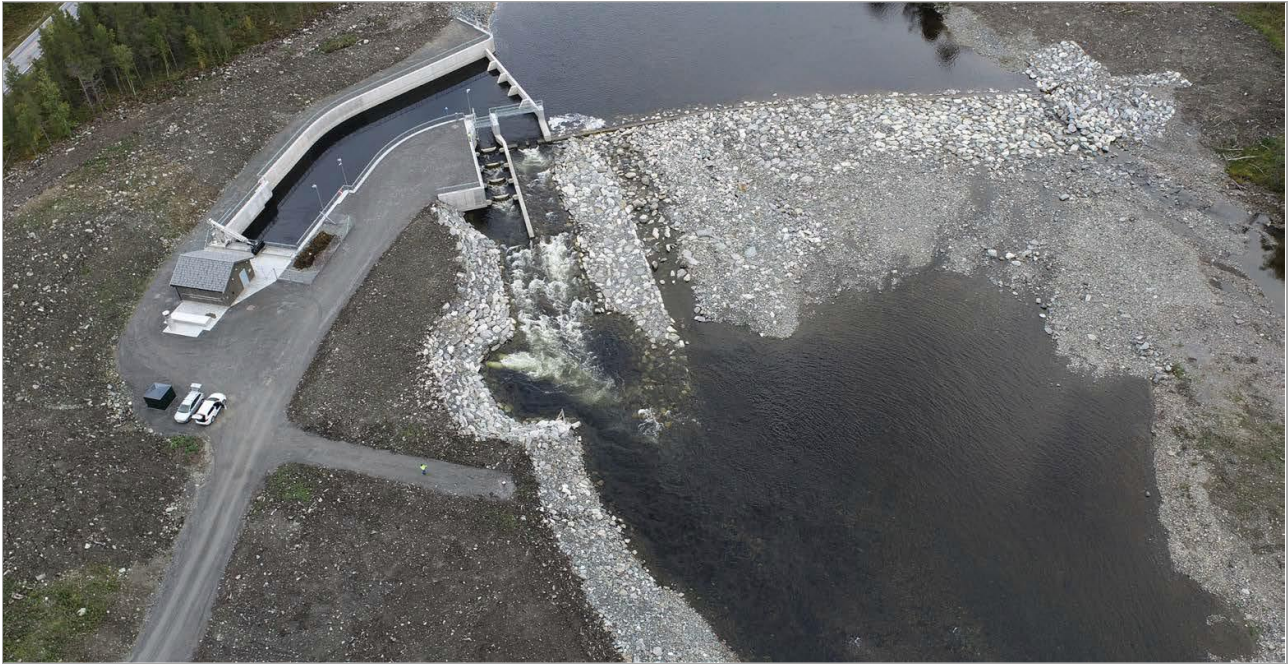
Figure 7.26 The Tolga hydropower plant, Hafslund (© Hafslund)
