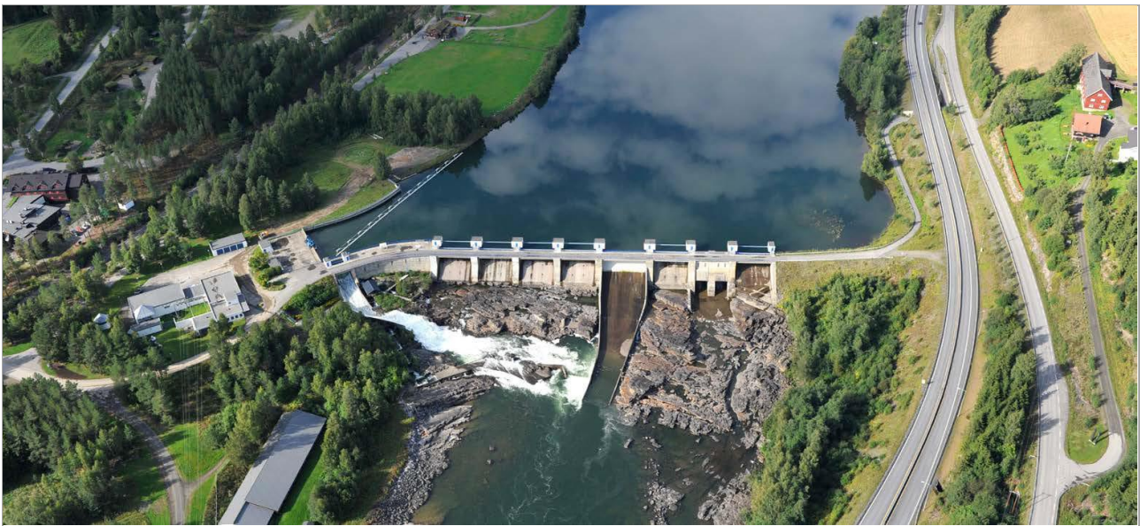
Figure 7.27 The Hunderfossen hydropower plant, Hafslund (© Hafslund)
