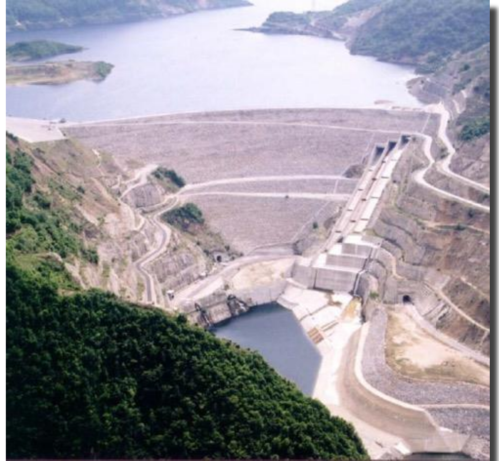
Thissavros Dam, Greece, 172 m
